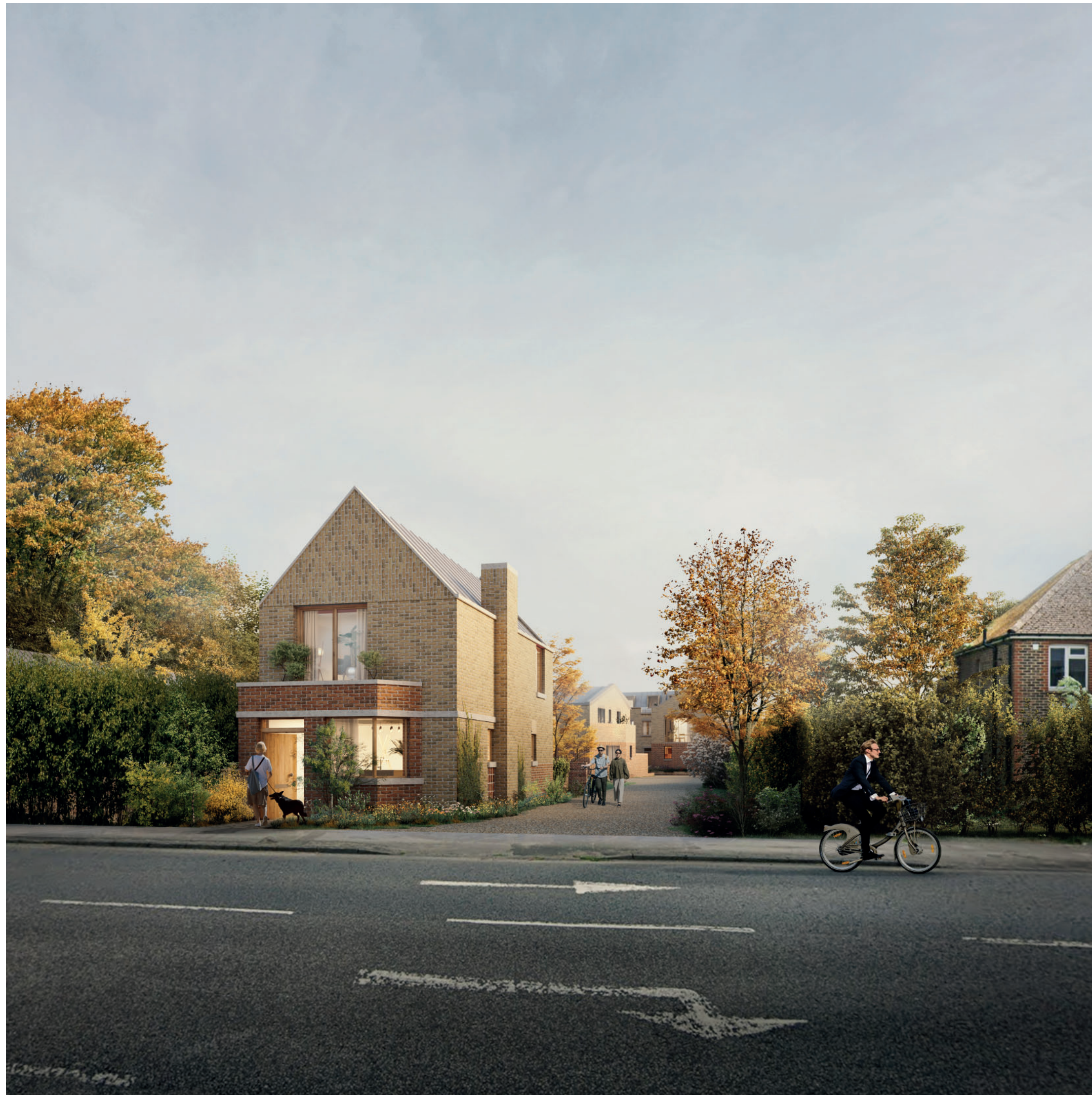
Proposed image of the front of the site along London Road.
