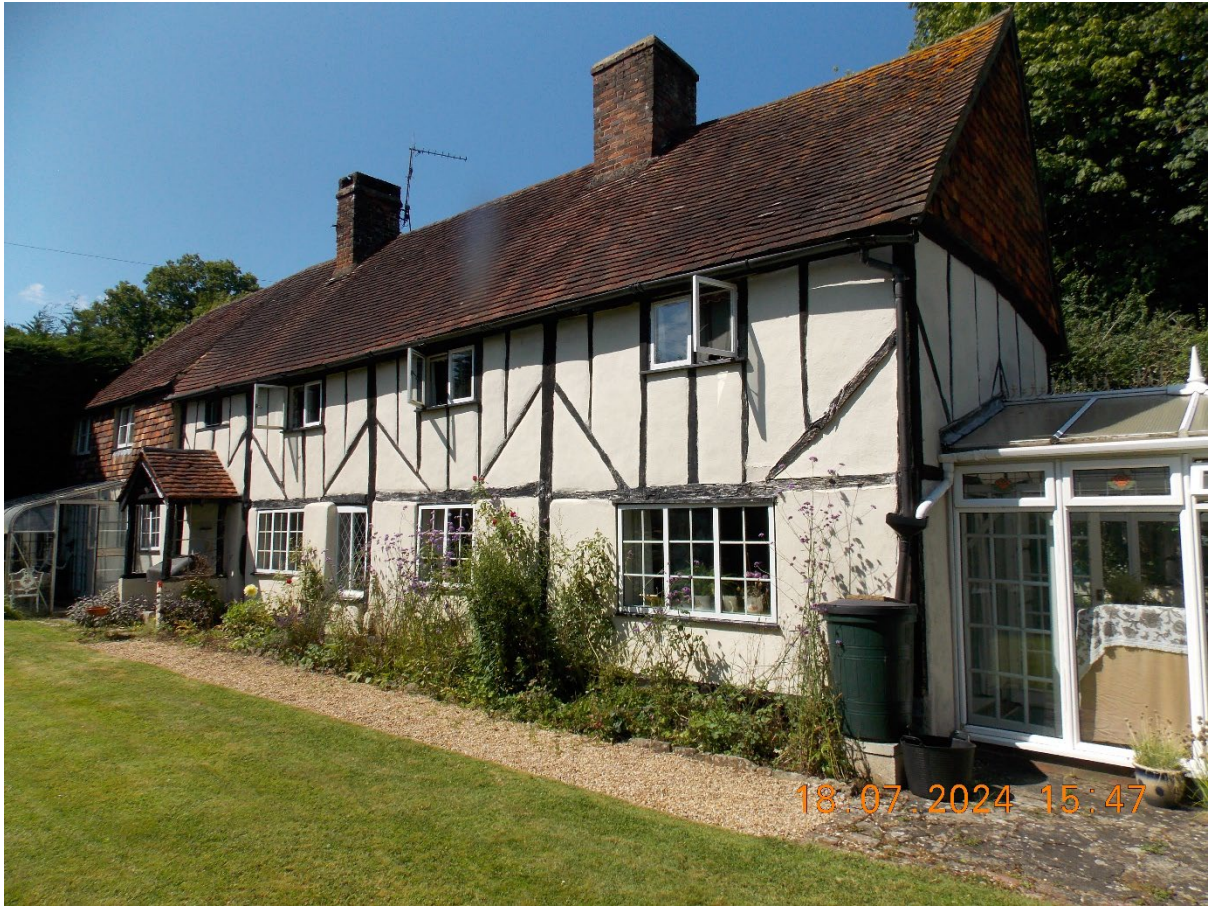
Fig 4. The listed building from the south-east.
