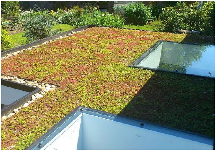
EXAMPLE OF SEDUM ROOF (Aesthetic, biodiversity & rainwater attenuation benefits)
