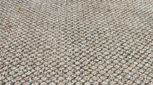
Cellular paving grid with decorative aggregate infill
