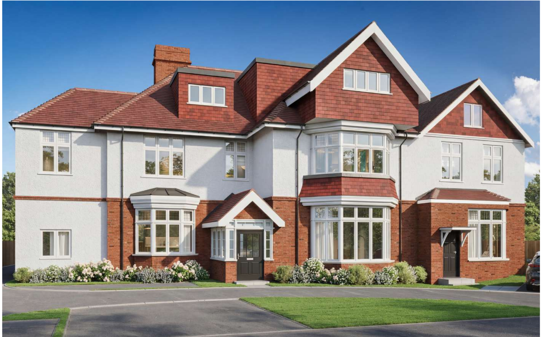
FLATS 1-7 GRANTLEY COURT — VIEW FROM YORK ROAD
