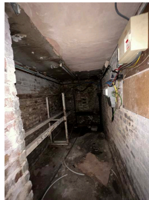
Image showing one of basements
