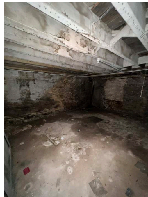
Image showing one of basements
