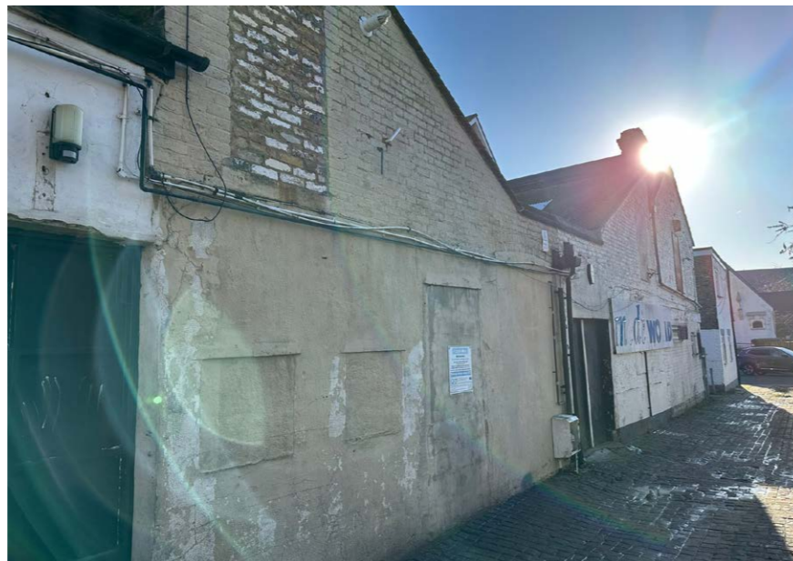
View of the rear elevation
