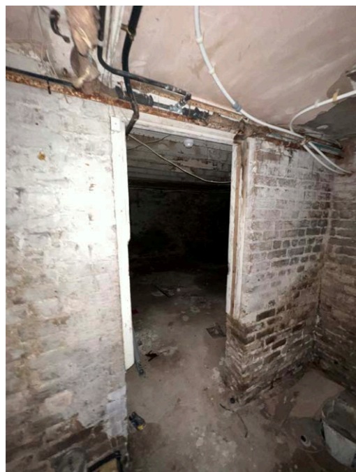
Image showing one of basements
