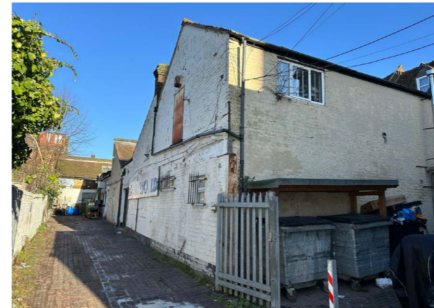
View of the rear elevation
