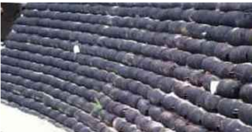
FLEX MSE vegetated wall system - CONSTRUCTION
