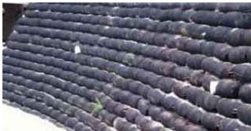
FLEX MSE vegetated wall system - CONSTRUCTION
