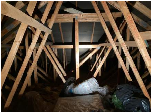
Centre of roof void
