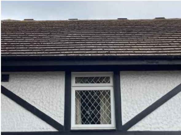
Ventilator tiles along ridge line
