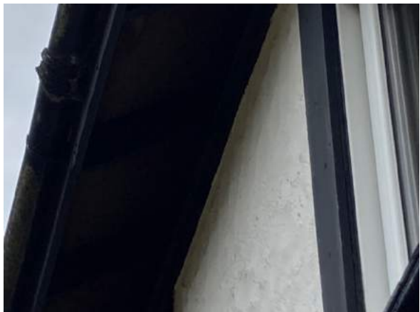
Wooden panelling along eaves
