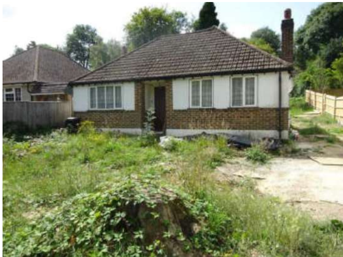
No.88 Caterham Drive (to be demolished)
