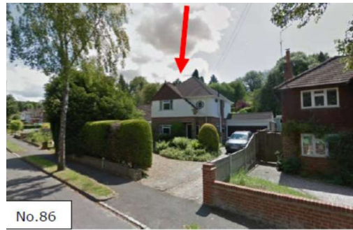
Figure 11: Photo of No.86 (to be retained)
