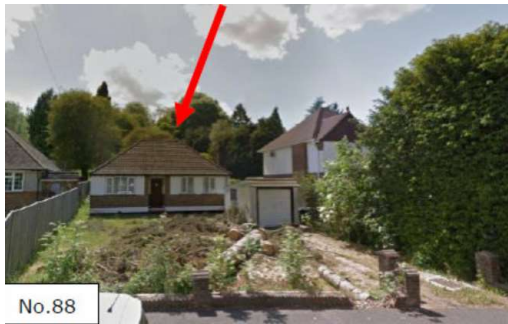
Figure 10: Photo of No.88 (to be demolished)
