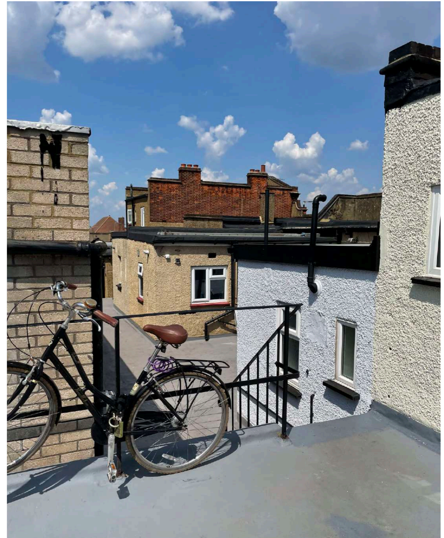
3.21 The existing development has a lack of cycle storage, which can be addressed in the new proposals
