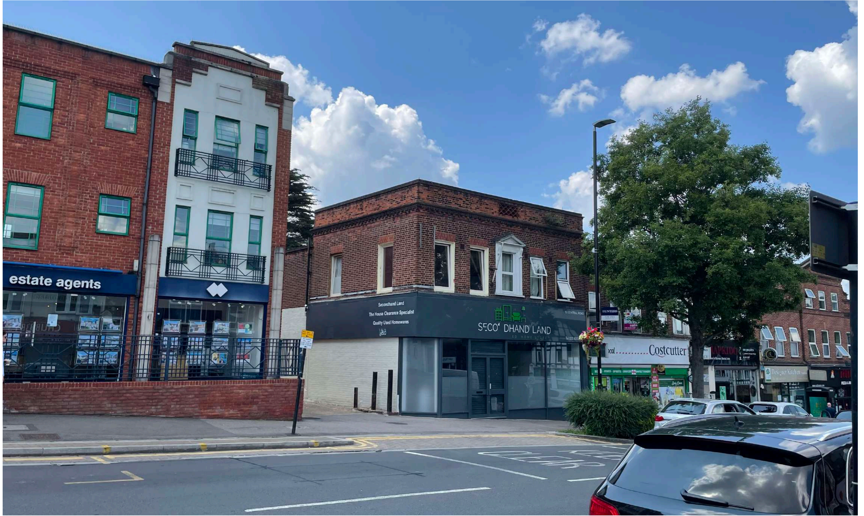
1.01. View towards application site from Central Road
