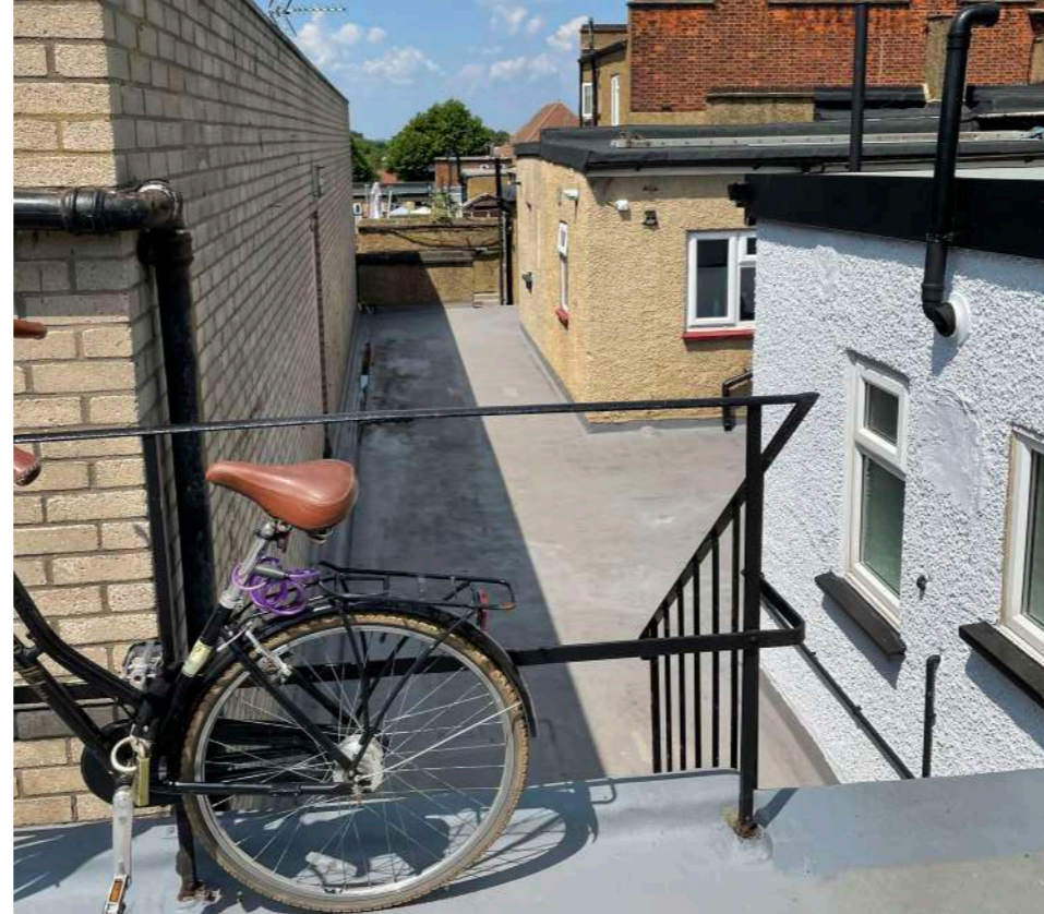
2.16. Existing roof access to adjacent residential units
