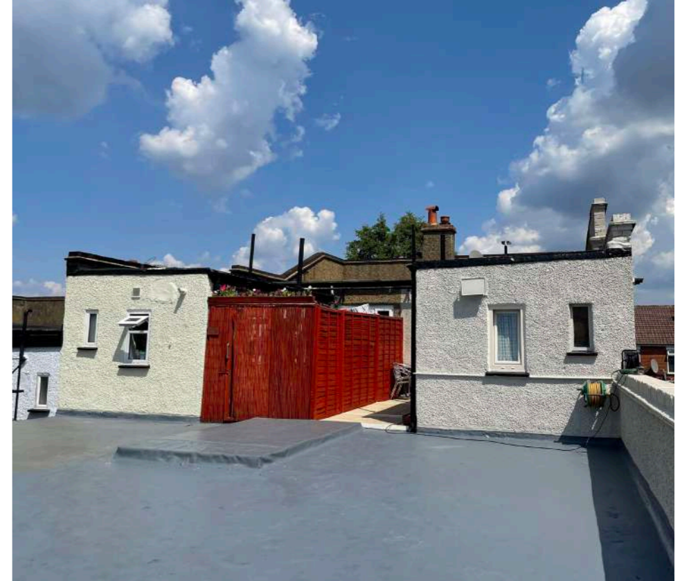
2.17. Rooftop view towards existing residential units on the site
