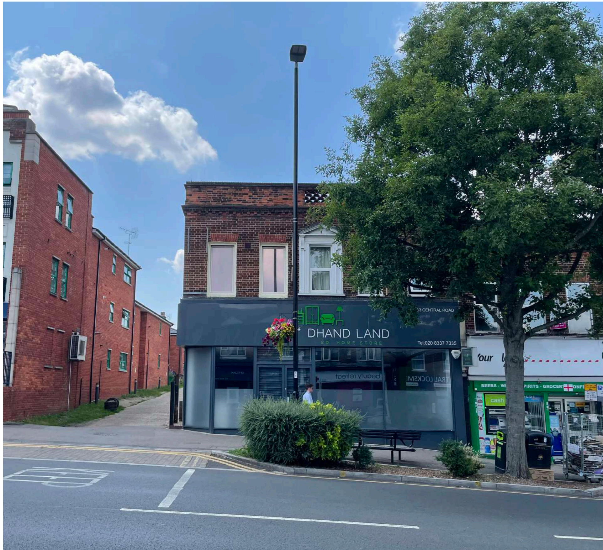
1.02. View towards application site from Central Road
