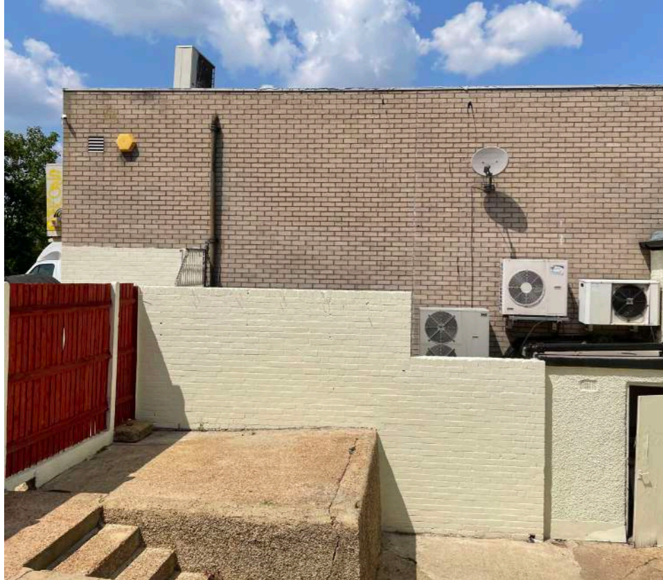
2.15 View of existing building yard
