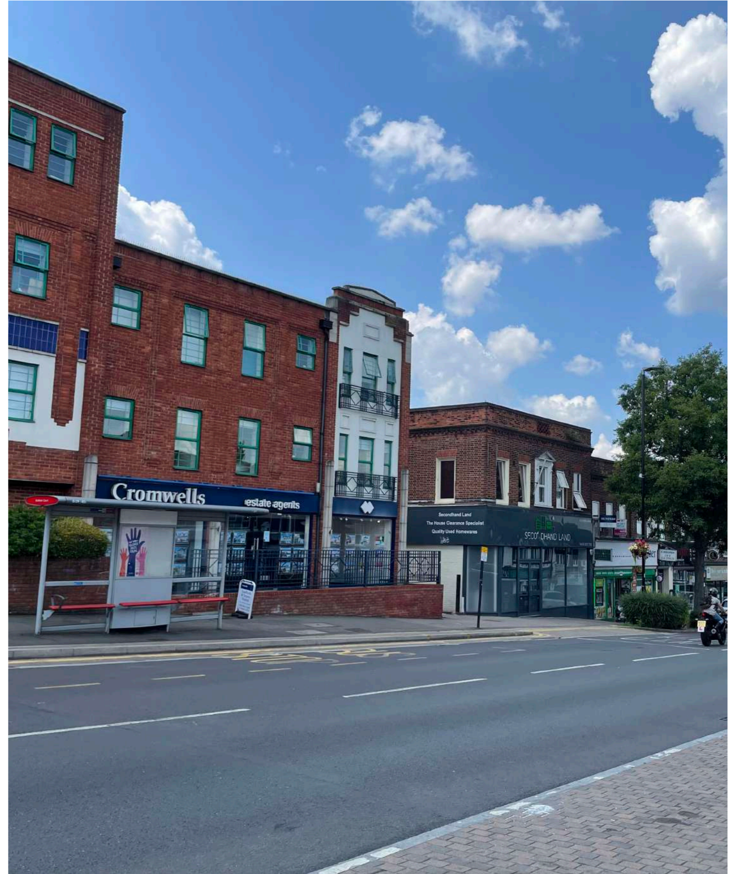
5.18. The site is within close proximity of local public transport links (such as the bus stop pictured).
