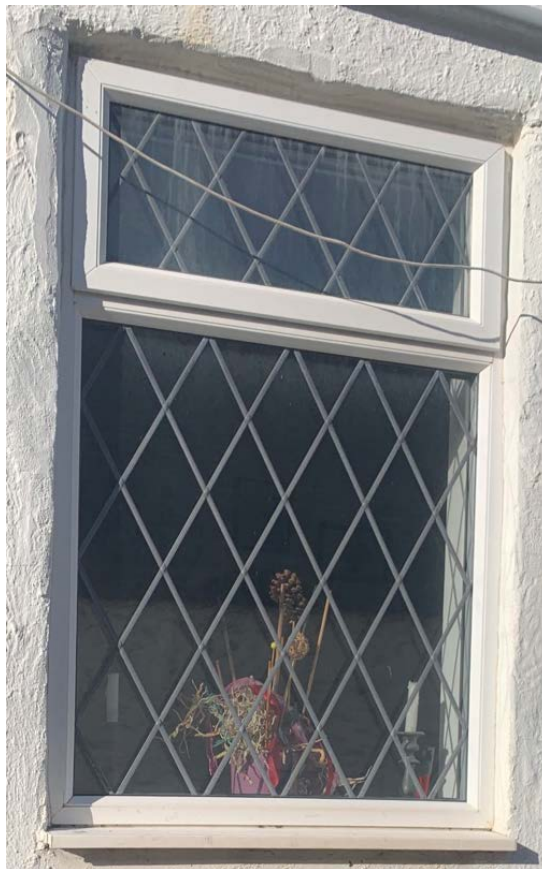
Figure 9: Window 7 as per Site Survey
