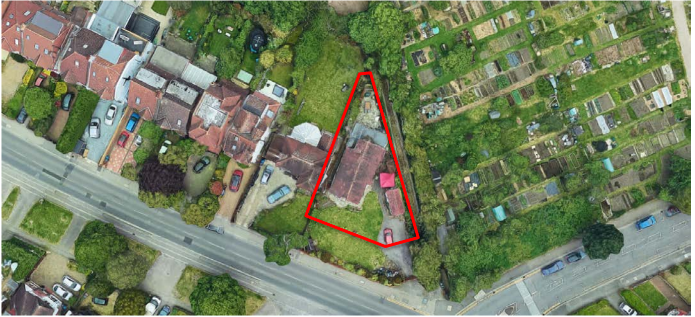
Figure 4: Aerial view of the site as existing.
