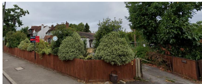
Figure 31. Street view of 260 Coombe Lane showing the shrubs at the front. Google Maps.
