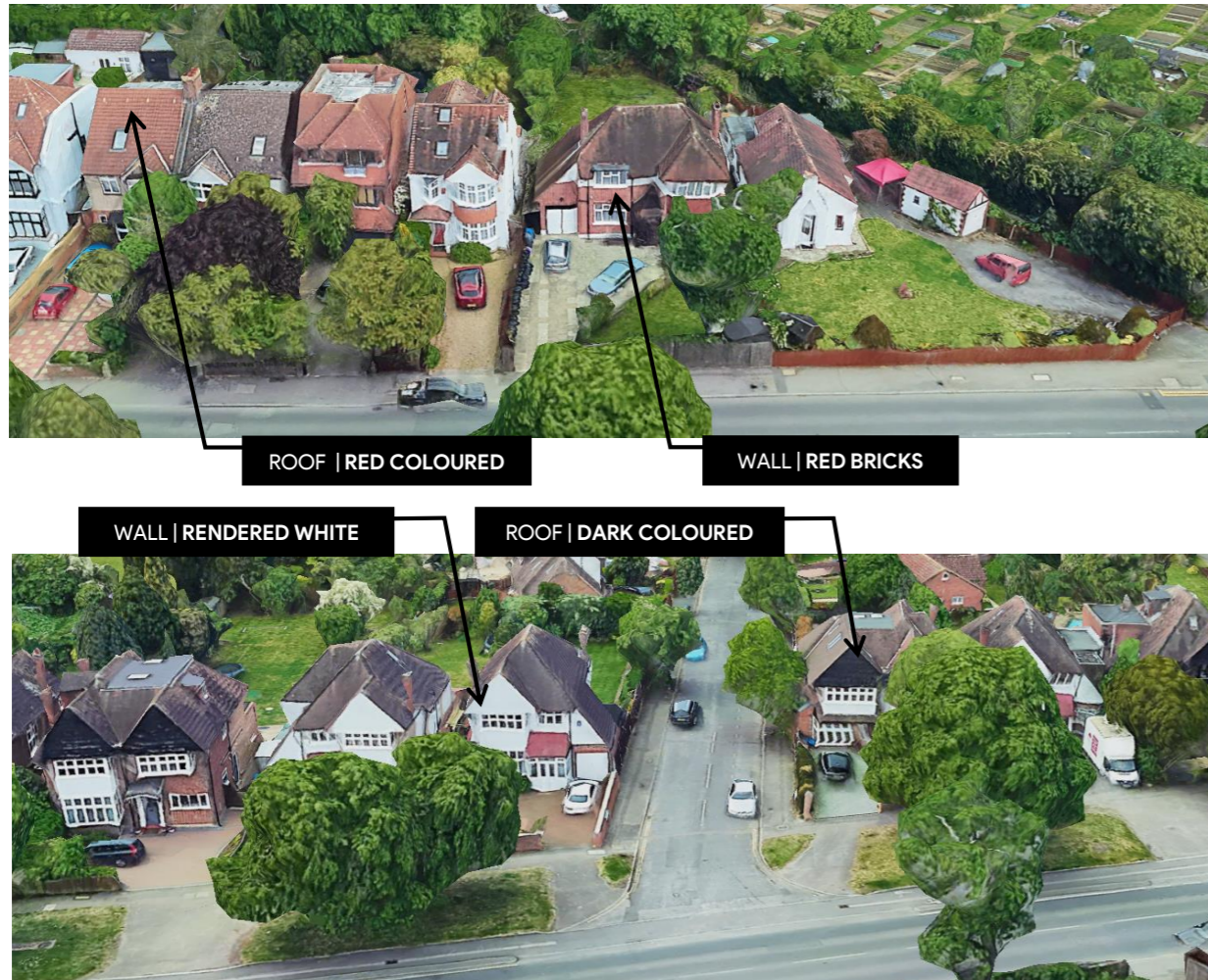
Figure 28. Aerial view of nearby properties pointing out similar material characteristics.
