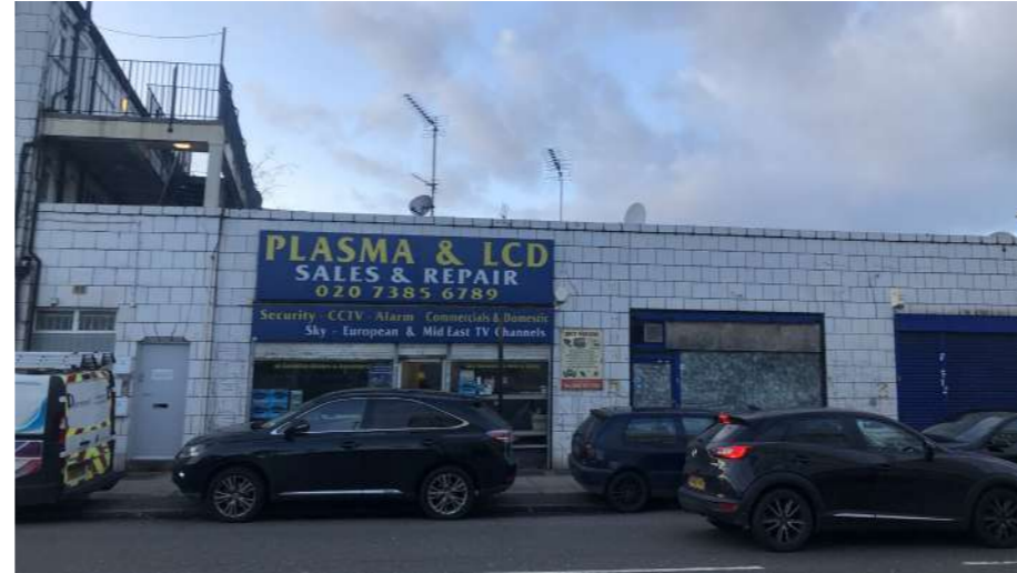
1. View on the site's building units 1,2 and 2C Image illustrates the current facade with front signage for the business unit in place as well shop glazed openings with shutters. Current premise is clad in matching tile to neighbouring building.
