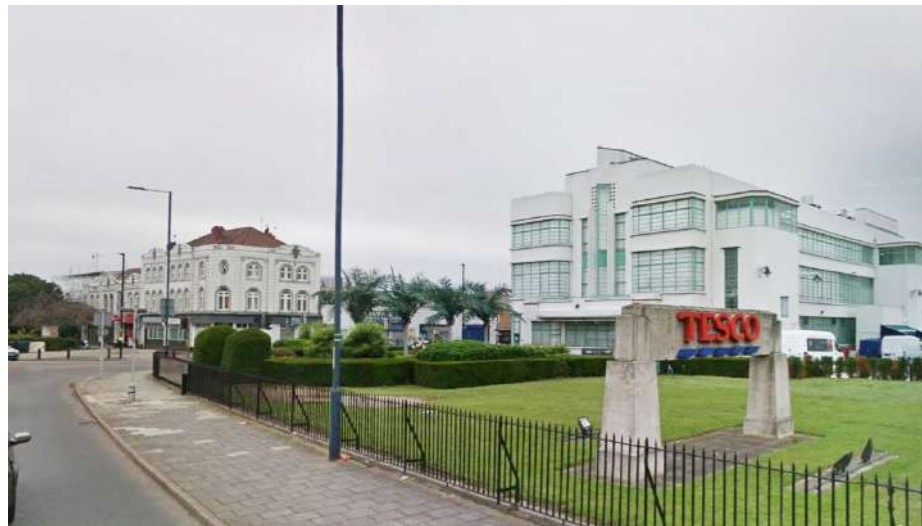
C. Forecourt piers, gates and railings to Hoover factory & other gates. Designation Type: Listing Grade: II
