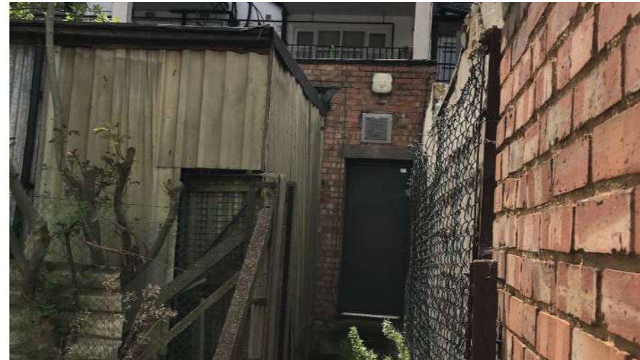
3. Shared access- rear entrance to ground floor premises of Lloyds Bank building.
