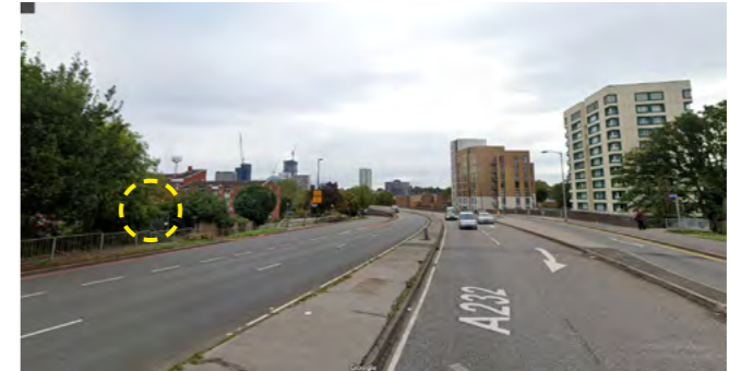
1 Arrival in car across Croydon Flyover, the skyline is defined by towers in East Croydon
