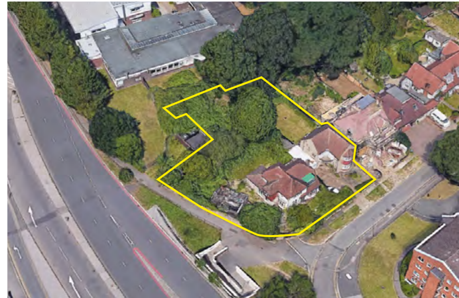
South-East Aerial View
