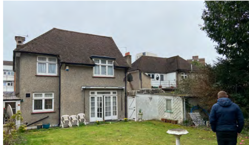
Rear of 3 Duppas Hill Terrace
